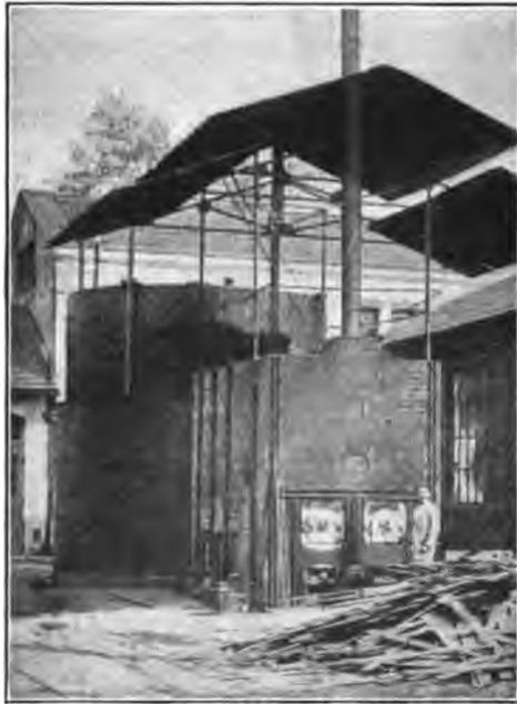
FIG. 100. — ASSEMBLY OF RICHE DISTILLATION GAS-PRODUCER.
